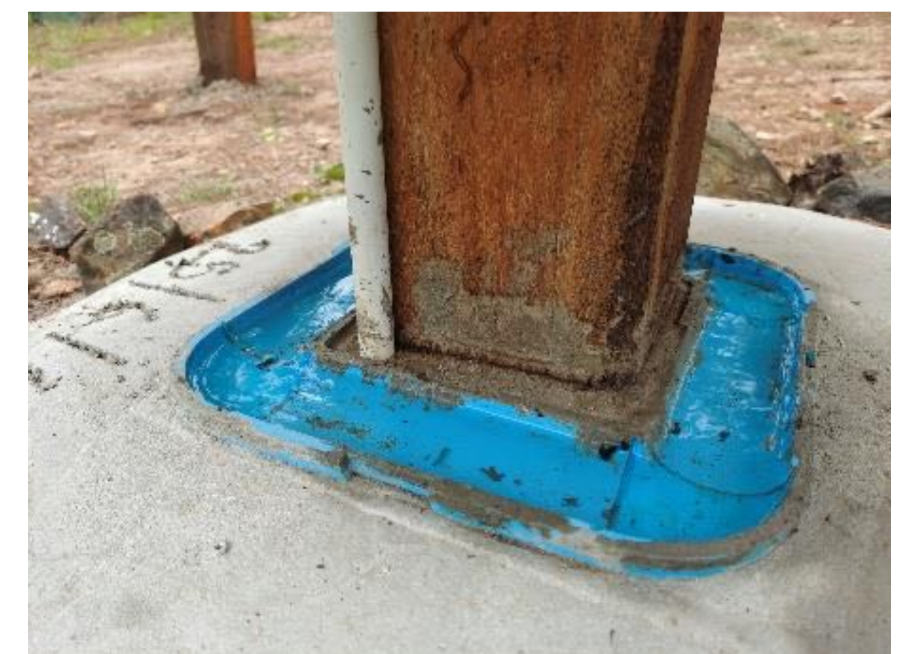
Motor Oil tray to protect insects and snakes
