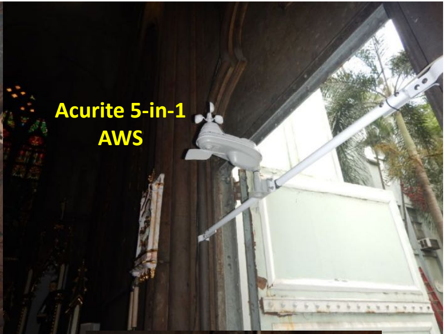
THVDR3 – Basilica's East Side Front Door
