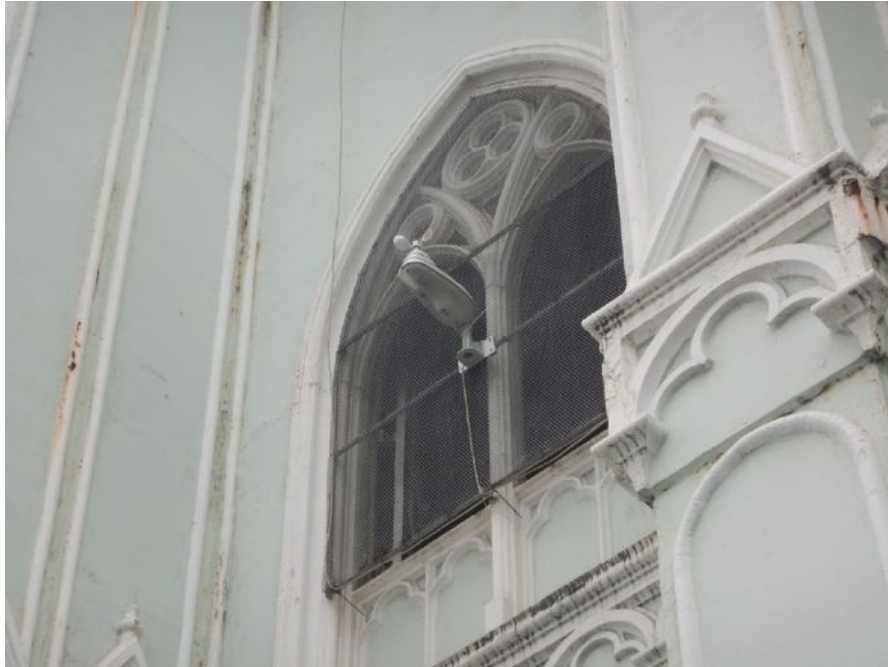
THVDR4 – Basilica's Right Tower, 1 Level Below Bell Tower
